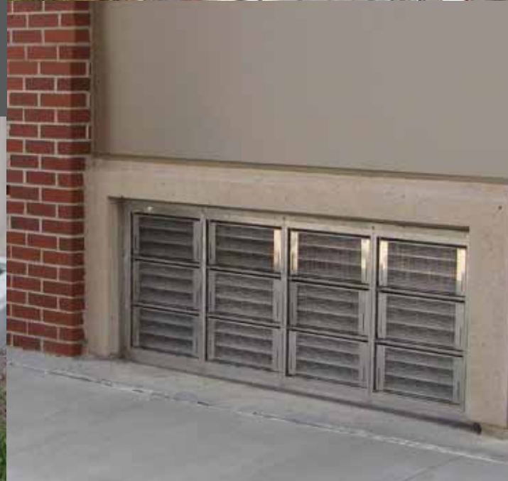
4 x 3 multiframe = 2,400 sq. ft. of flood protection
