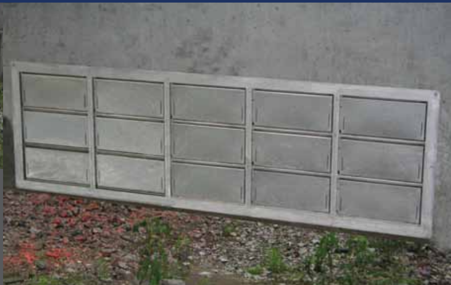
5 x 3 multiframe = 3,000 sq. ft. of flood protection
