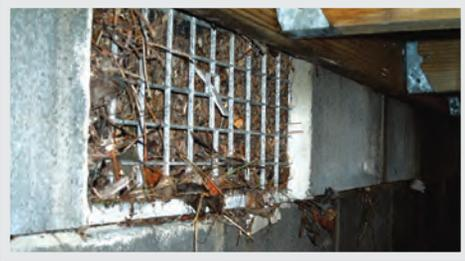
**Typical air vents will clog with debris** during a flood event. A 3" opening must be maintained at all times in accordance with ASCE 24-05 for any flood opening to be accepted.
