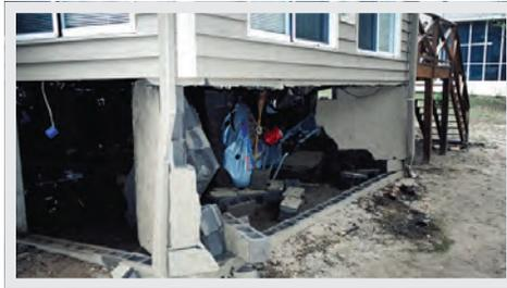
**Structural damage is caused by the build up of hydrostatic pressure** when a flood occurs. Standard air ventilation devices that have detachable solid covers are non-compliant because it is assumed the homeowner will cover the vent.
