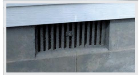
**Air vents that can be closed manually are not compliant** unless they are "permanently disabled in the open position," according to FEMA's TB1. Even if broken into the open position, these vents provide little to no area to allow for debris to pass through.
