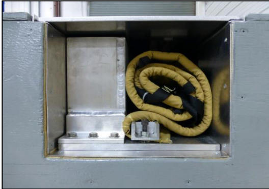
Packed in Trench
