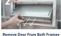
With the vent flange facing you, rotate the bottom of each vent door outward and slide out of frame.
