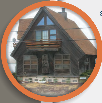
First Smart Vent installation in Avalon, NJ. 1999
