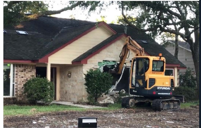
Yelovich Residence Demolition
